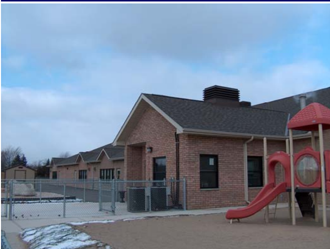
Photo of the addition to St. Anne Catholic School in Blenheim, following the school's consolidation with the former St. Mary Catholic School.
